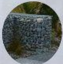
Landscape treatment including planting, gabion baskets, rock placement, exposed aggregate treatments and lighting
